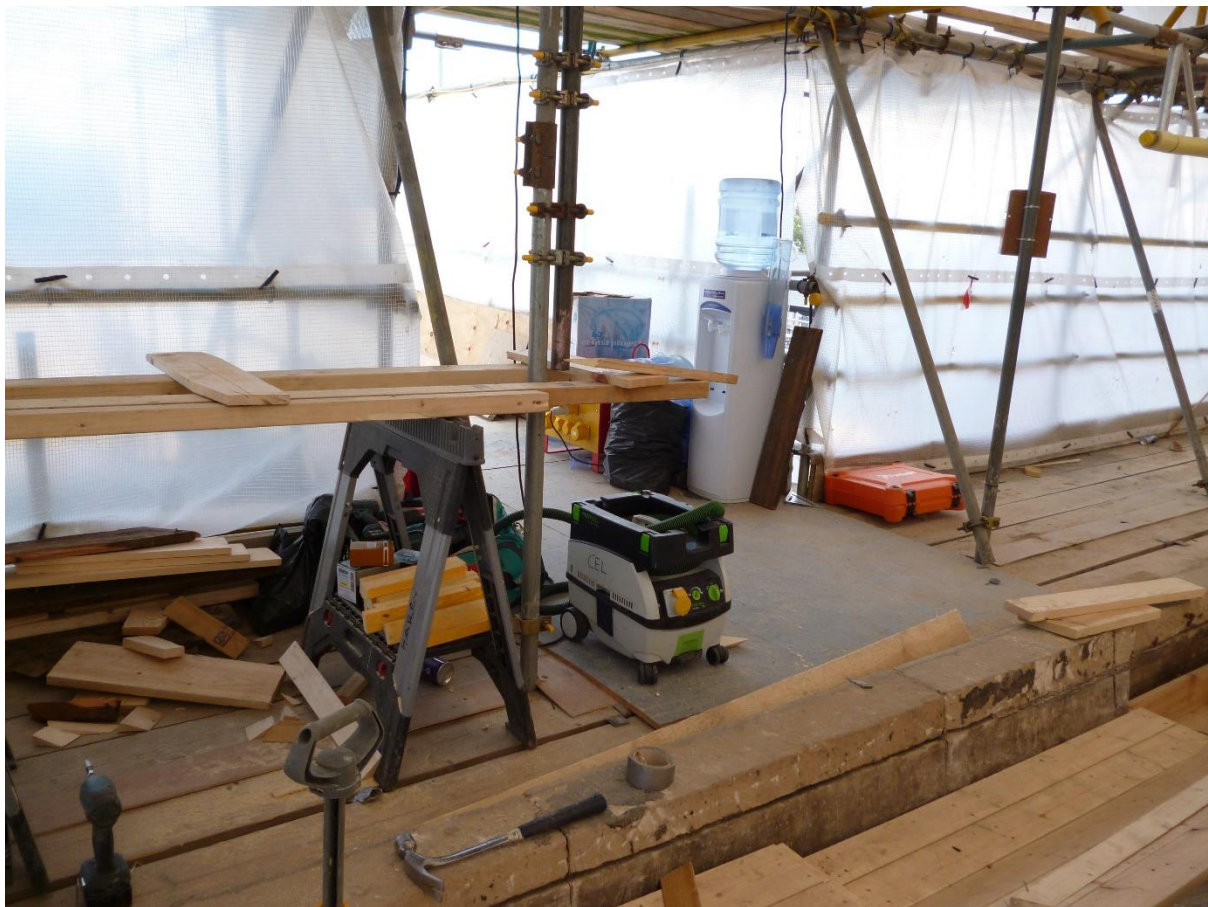
Portable dust extraction is increasingly used in construction to manage dust exposures
