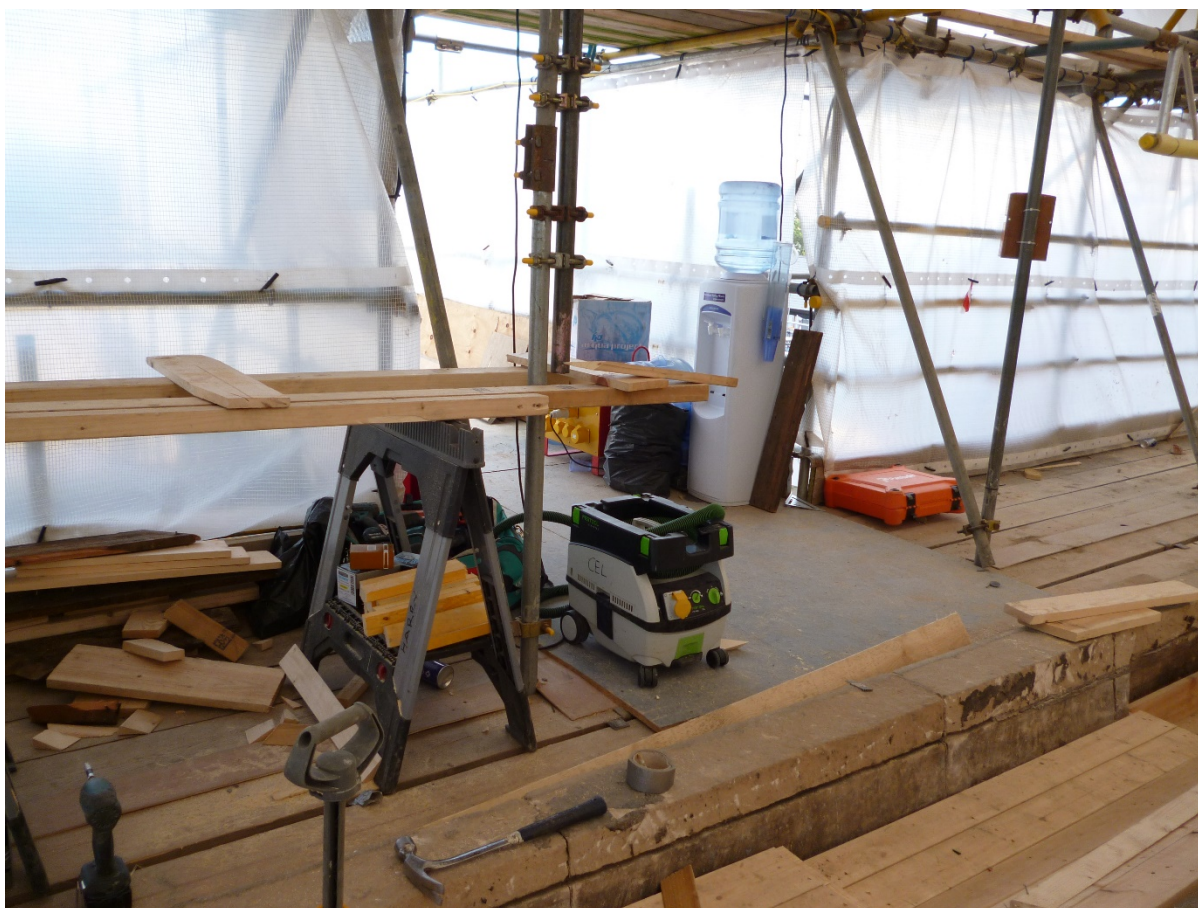
Figure 1 Portable dust extraction is increasingly used in construction to manage dust exposures
